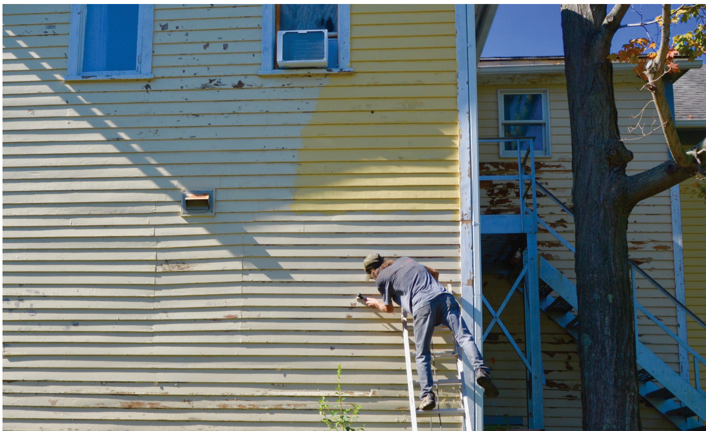
Orchard House receives a fresh coat of paint.
